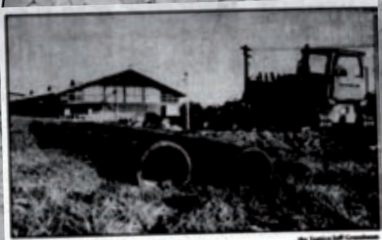
Construction is underway for Brandeis' new athletic center.
