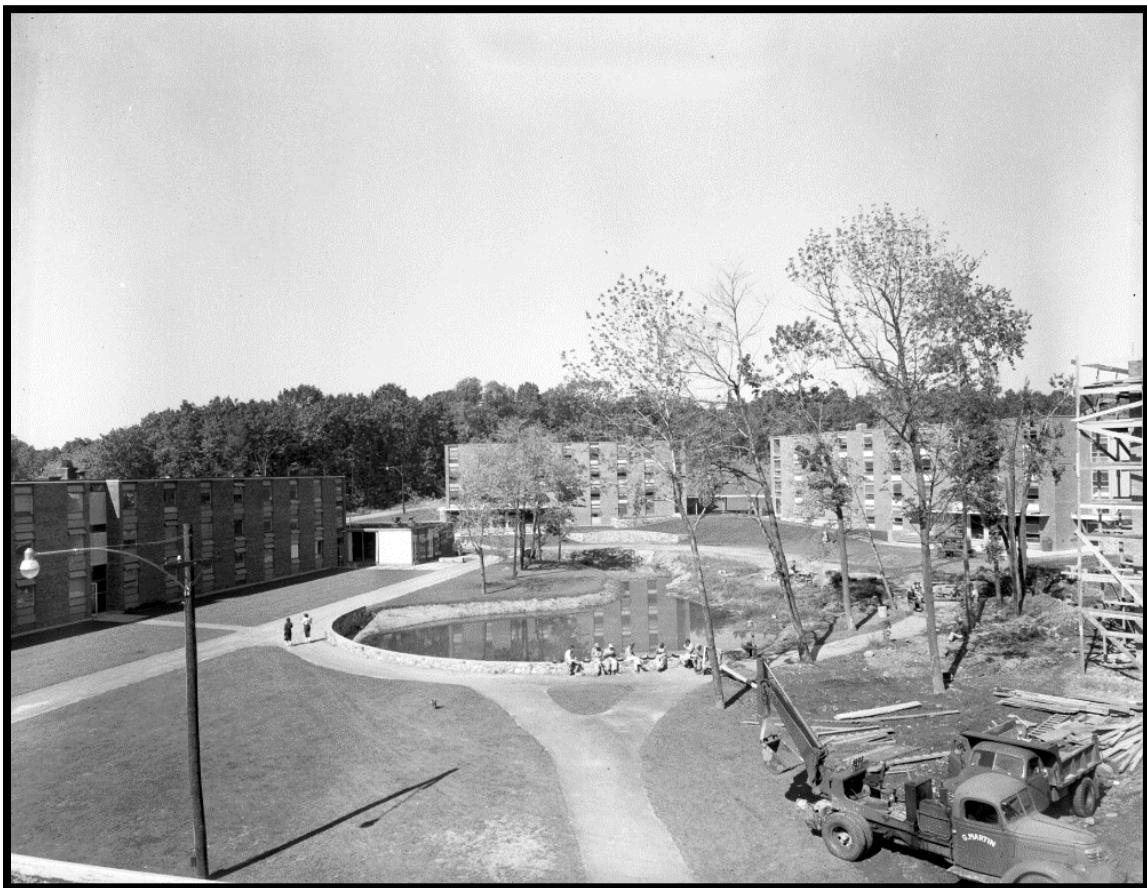
The "New" Girls' Dorms – Hamilton A, B, C – in construction
